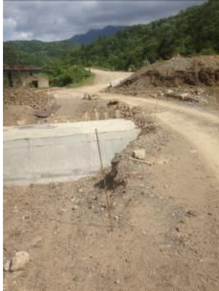
Deep excavation without hard barrier, warning signs KM16
