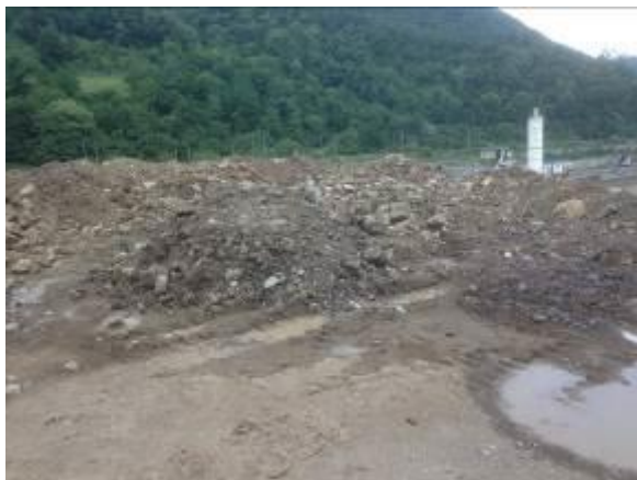
Spoil stokpile and heavy equipment working without flagman
