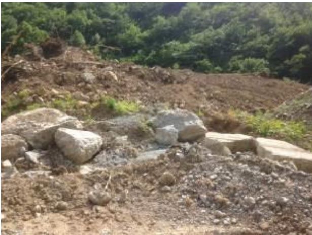
Mixed spoil, vegetation roots and concrete debris
